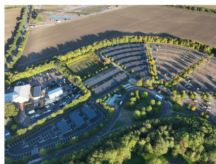
Figure 3: Babraham Park & Ride solar panel installation (Phase 1). Credit: Cambridgeshire County Council.
