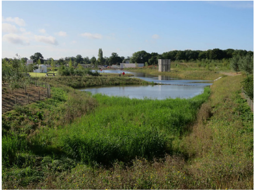
↑ Lagoon constructed at the Eddington site, as part of the nature-based solutions to flood attenuation and rainwater harvesting scheme, which contribute to achieving water neutrality. Credit: Hugh Venables.
