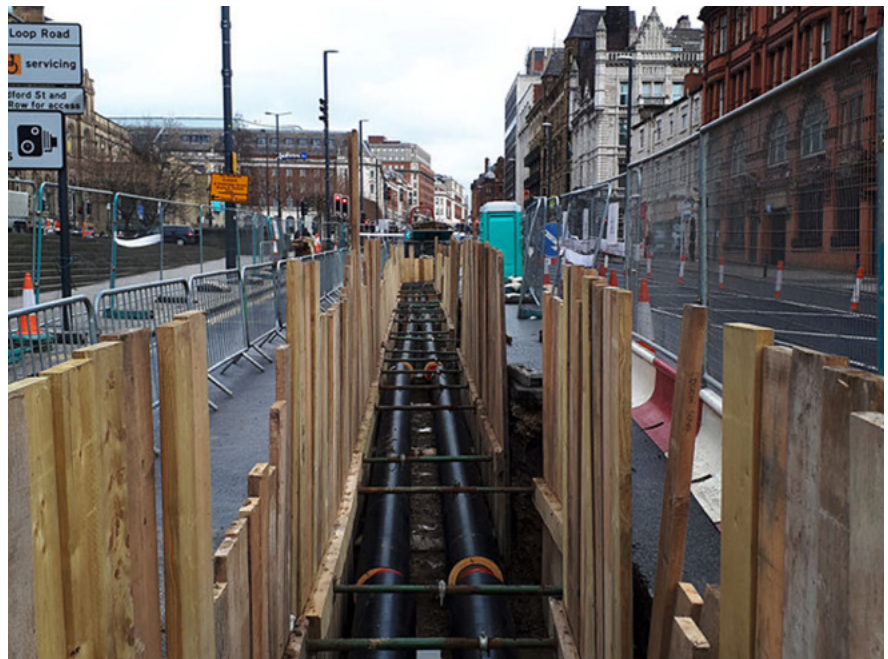
↑ District heating pipes being installed in Leeds, as part of the PIPES scheme, serving civic buildings in the city centre. Credit: Stephen Craven.
